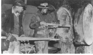
Sparrows Point workers cleaning a furnace by removing “slag,” a toxic by-product of molten metal, sometime in the 1940s. COURTESY OF THE DUNDALK-PATAPSKO NECK HISTORICAL SOCIETY
